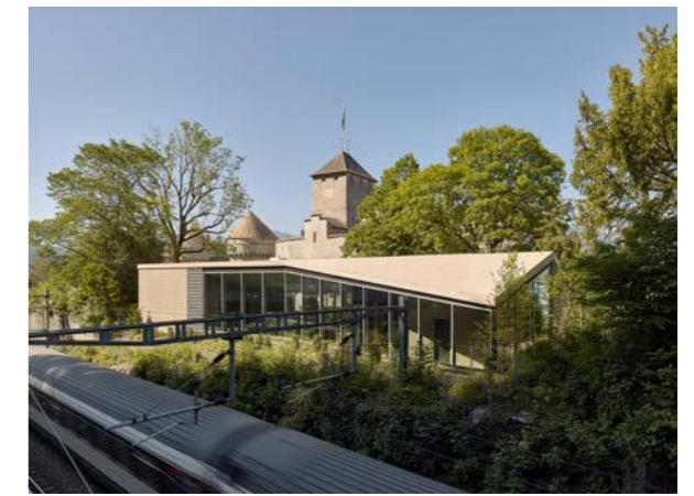
Jardin Anglais Cafe Pavilion. Chamfered roof forms add visual interest to linear built form
