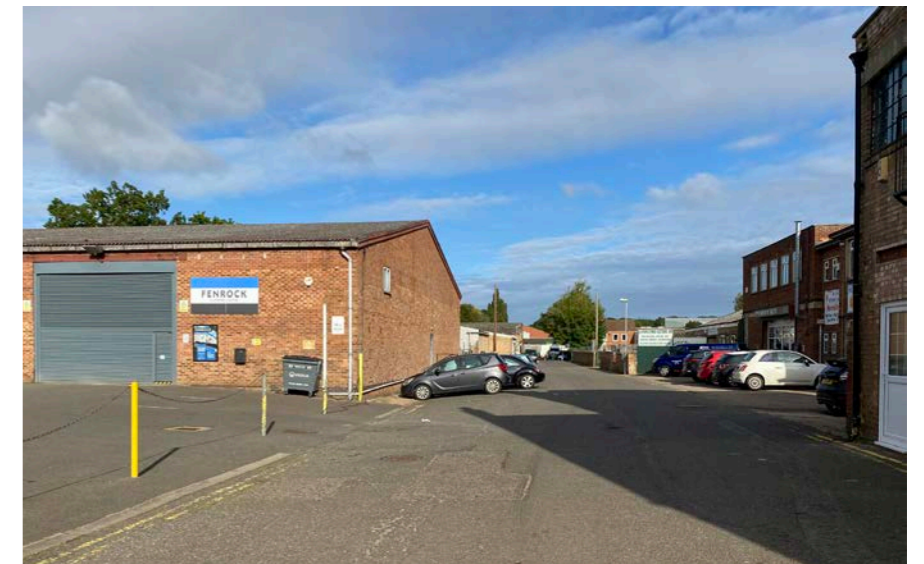
View of the Chapel Road housing site - currently under multiple ownerships
